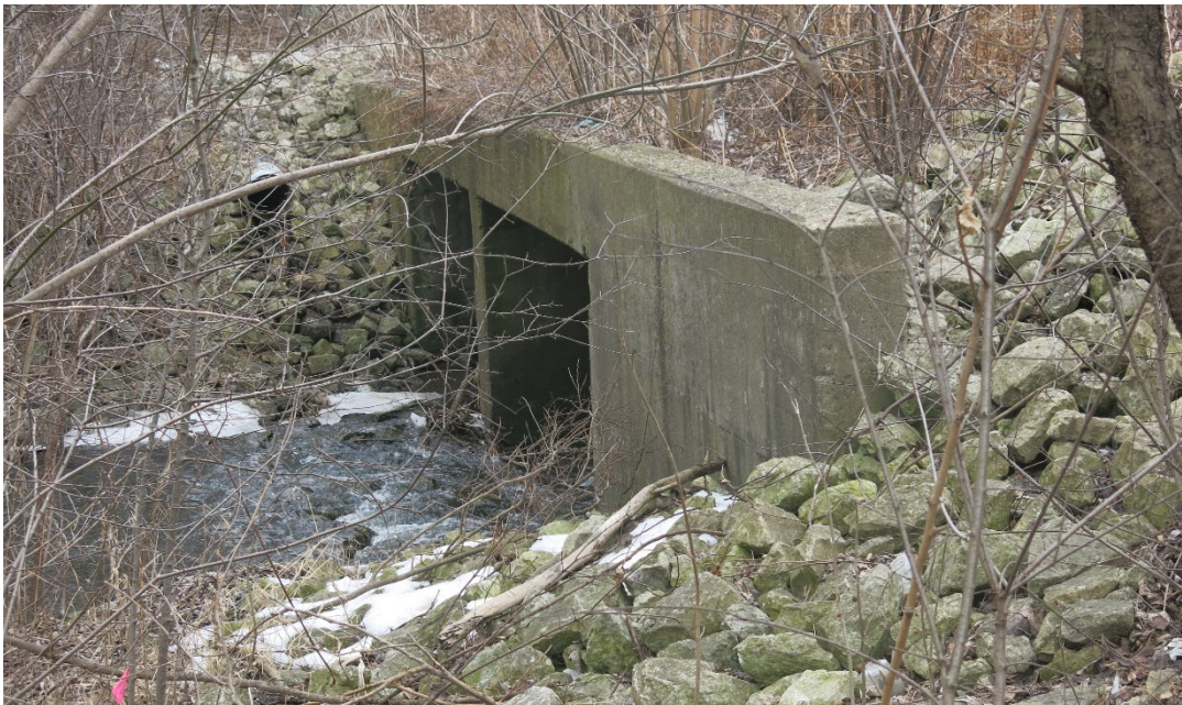
Photo 1: Existing Palatine Road culvert upstream face looking southeast
