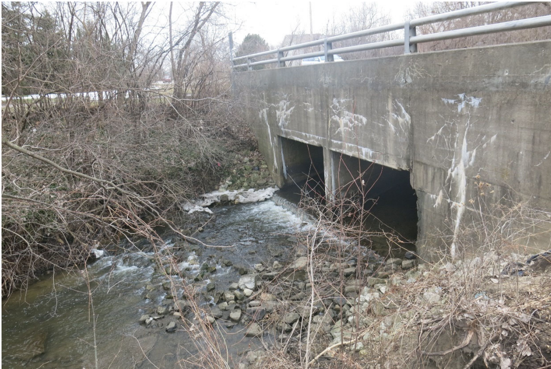
Photo 4: Downstream face looking northwest
