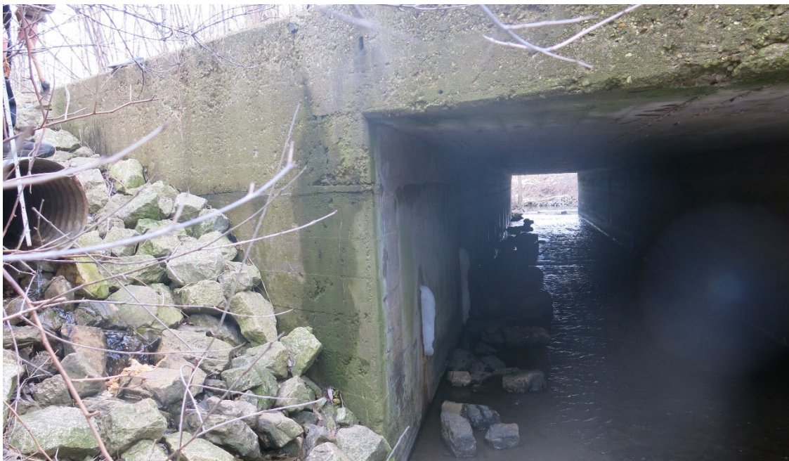
Photo 3: Upstream looking south
